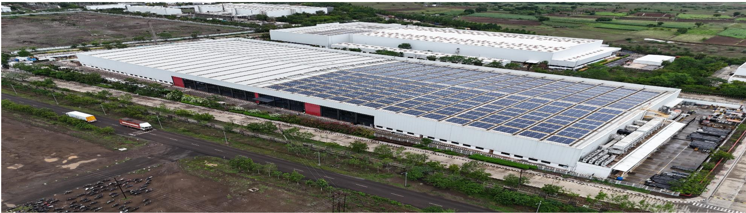
Size of Plant is 7 Acers
